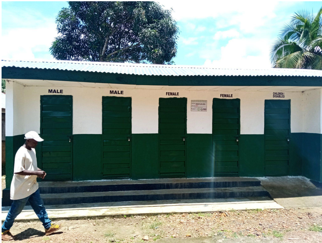
Figure 4. Block of community toilets with five squat holes separated by gender, age, and physical conditions in Matakan village, Niawa Chiefdom.
